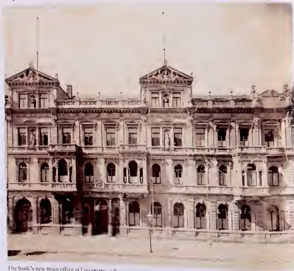
The bank's new main office at Luisenstrasse 9
